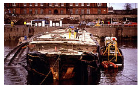
City of Adelaide being raised at Govan in 1992
